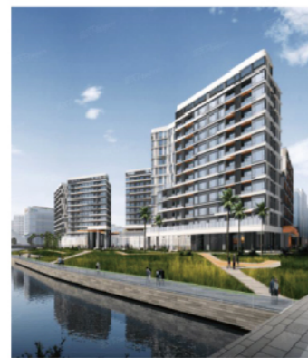
深圳会展湾云案广场 Shenzhen Convention and Exhibition Bay Cloud Case Plaza
