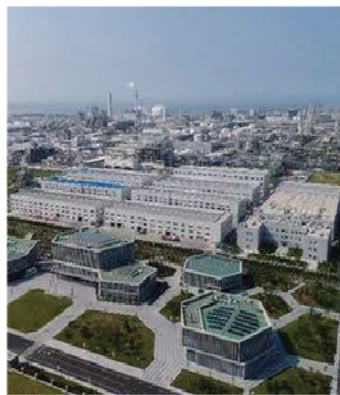
万华化学集团宁波项目 China Mobile anti-static flooring centralized procurement project
