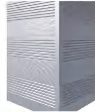
External corner joint
