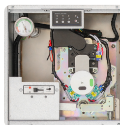
Figure 2-2 Load switch operating mechanism
