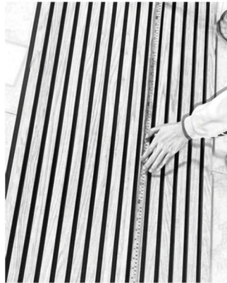
② Measure the wooden slat acoustic panel
