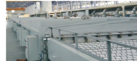
镀膜流水线 Continuous line
