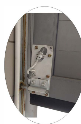
★ 可调底端支架，再也不用为了松紧一下钢丝绳而把整套门的扭簧松掉，拧拧螺丝，轻松搞定 ★ Adjustable bottom supporter, in order to no longer have a wire rope and the elastic torsion spring loose set of doors, screw, easily
