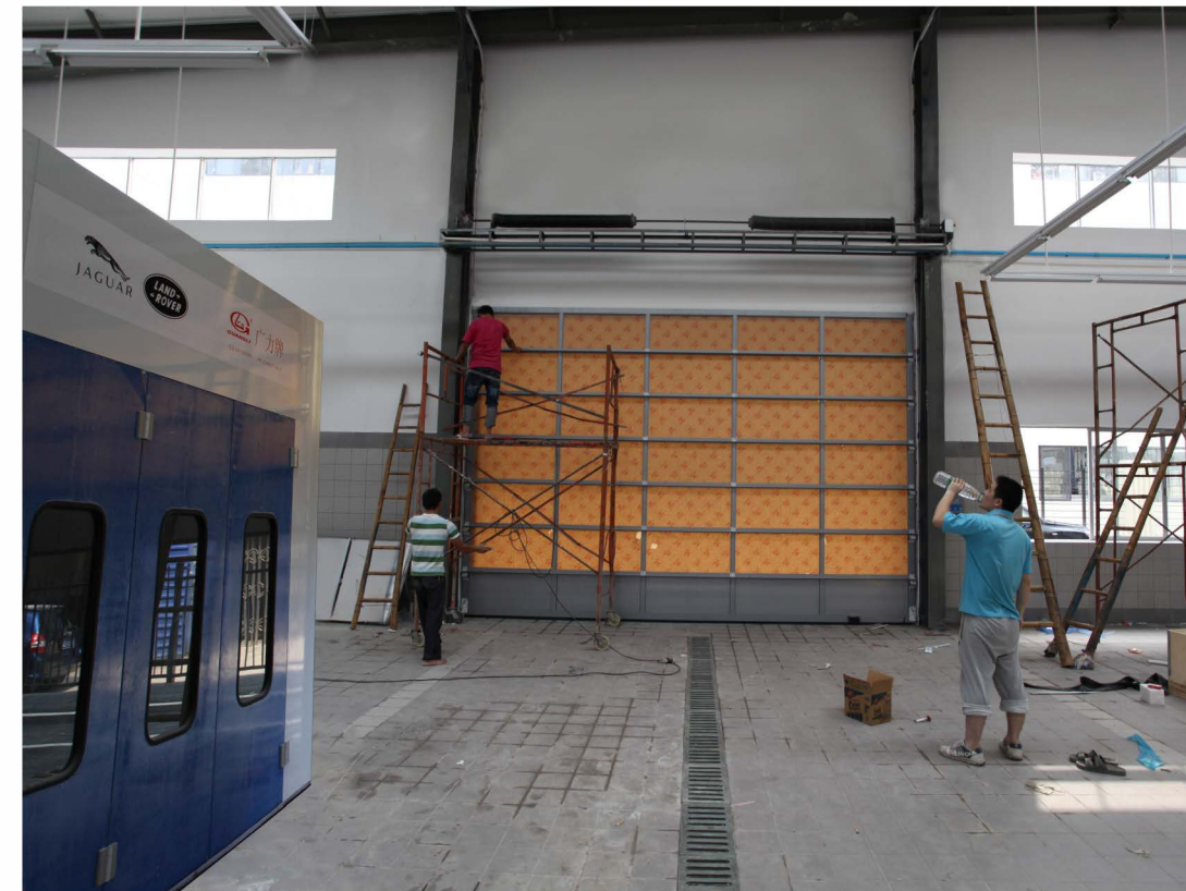
★ 铝合金透视门在捷豹4S店的安装应用 ★ Install the application of aluminium alloy doors in perspective of Jaguar 4S shop
