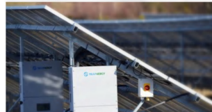
Inverter for reverse power transmission
