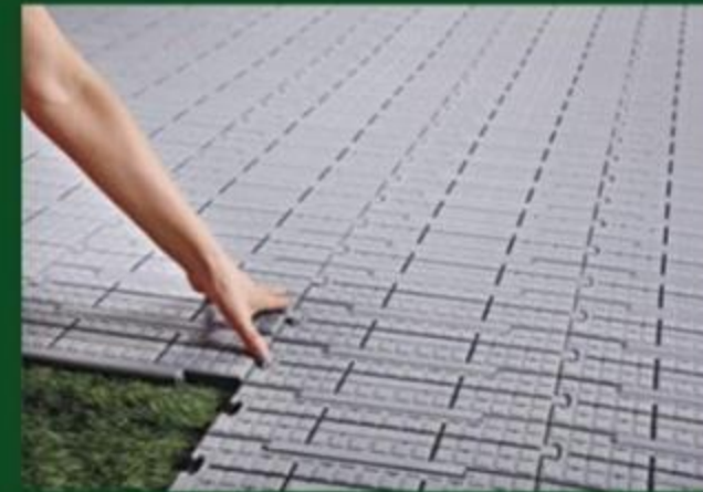
4. Press the pin to snap into the floor beside by thumbs or little wood hammer
