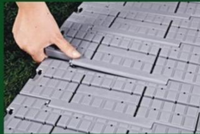
3. Connect the flooring with the pins one by one
