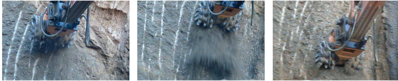
Milling and excavation of Hutubi tunnel
