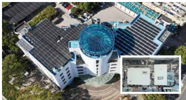
| Subdistrict Office in Shanghai, China 200kW
