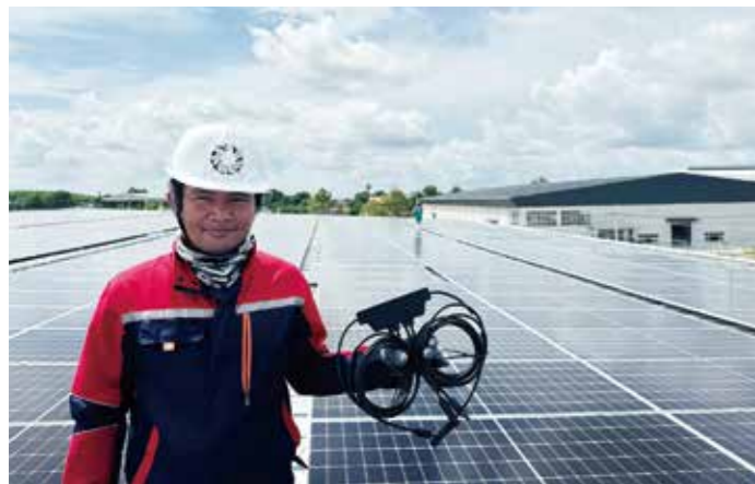
| Tool Factory in Rayong, Thailand 400kW
