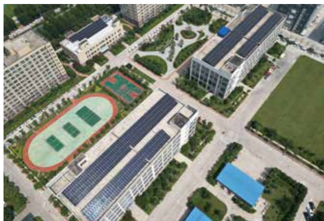
| Shijia Electric Factory in Henan, China 562.84kW
