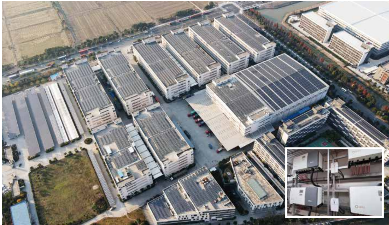
| MG Stationery in Shanghai, China 5.5MW
