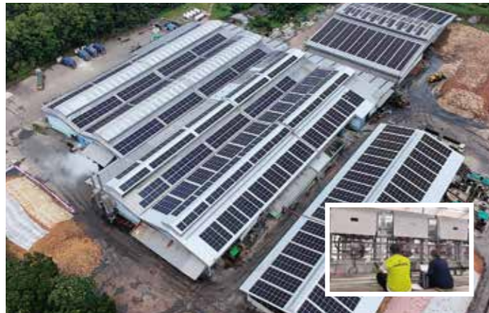
| Rubber Factory in Krabi, Thailand 2MW
