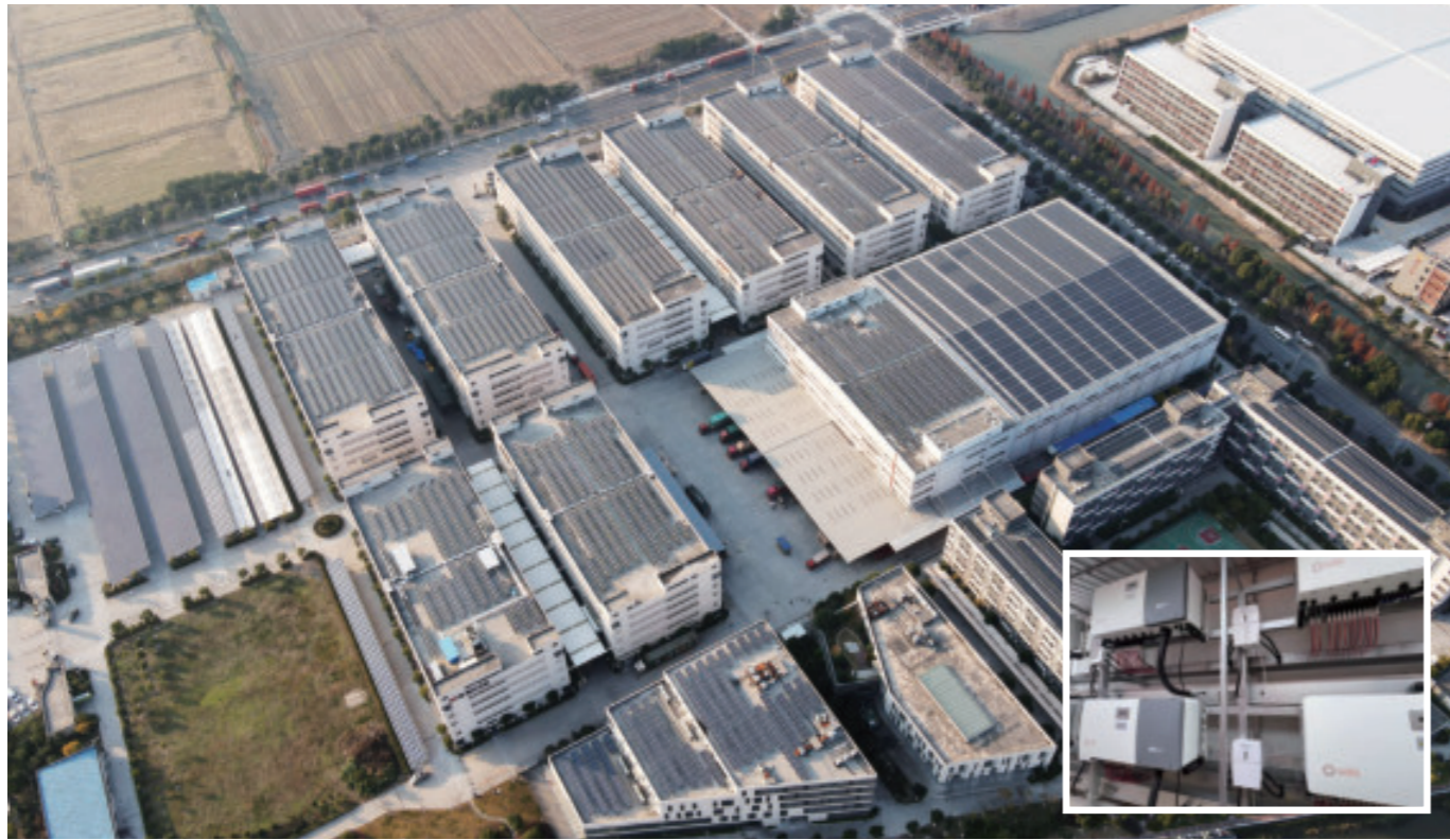
| MG Stationery in Shanghai, China 5.5MW
