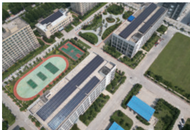
| Shijia Electric Factory in Henan, China 562.84kW
