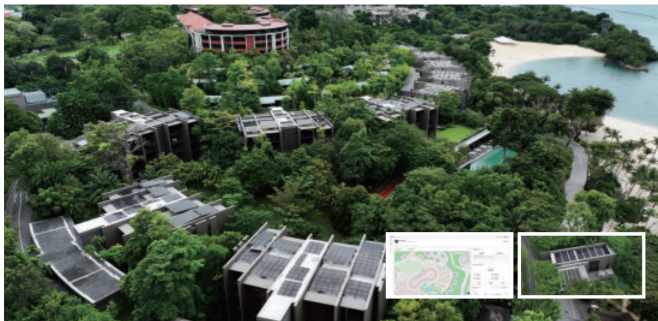
Capella Resort PV Project in Singapore 249.15kW
