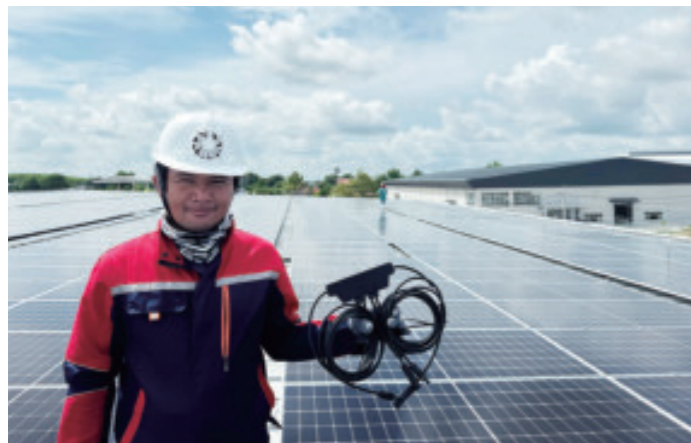
| Tool Factory in Rayong, Thailand 400kW
