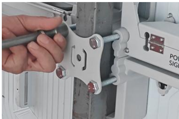
Lock connecting plate
