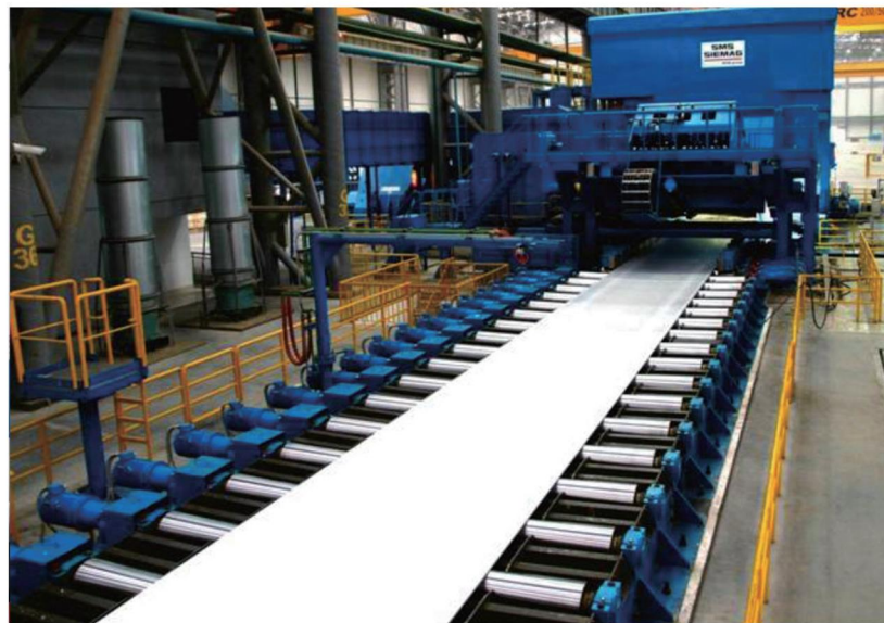
Hot Rolled Production Line 热轧线
