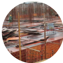
15 Building Bamboo Plywood
