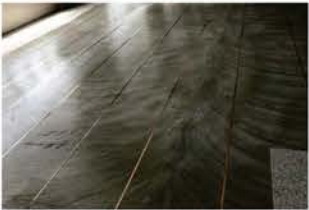
铺设铜箔 Laying copper foil
