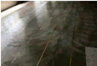
铺设铜箔 Laying copper foil
