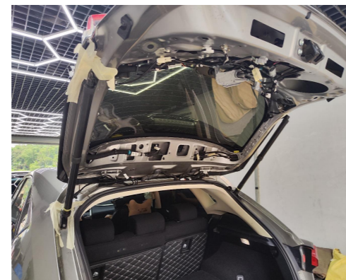
8. Install the electric struts, L on the left R on the right (the first letter of the strut code), making sure the ends with wiring harnesses are on the car body.
