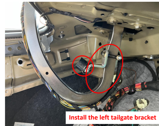
8. Install the left tailgate bracket and provided bump stop. For the right hinge, only replace the bump stop.
