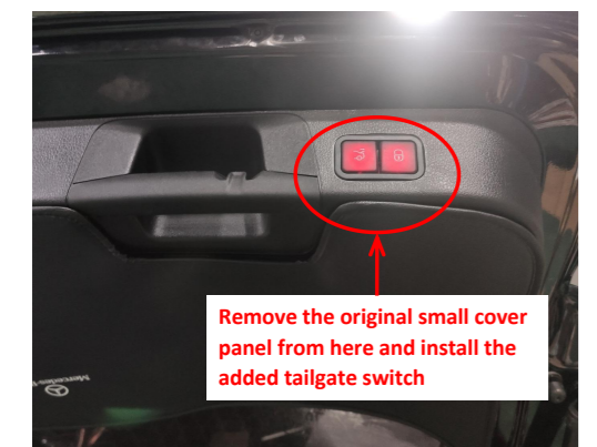
27. Install all trim panels back and install the added tailgate switch. (Check whether the buttons can bounce back normally. If there is any interference, use a knife to scrape the interfering part.)
