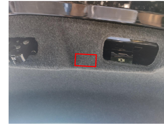
25. Stick the hole template to the indicated position on the trim panel and open a hole for the added tailgate switch (as close as possible to the lower edge of the trim panel).
