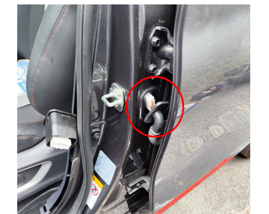
26. Connect the plugs of the power harness to the B-pillar signal plugs.
