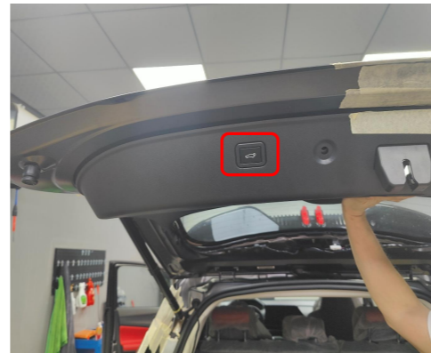
29. Remove the original small panel and install the added tailgate switch connect the plug of lock signal harness with it and reinstall all trim panels.
