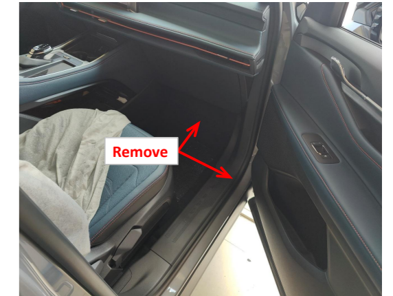
1. Remove the front passenger side trim panel and door sill panel. The fuse box is located behind the door sill panel.
