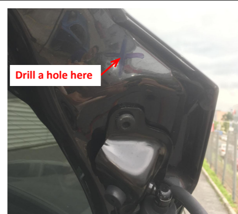
18. Drill a hole at the indicated position with a \phi 21\text{mm} drill bit and do the same on the other side.
