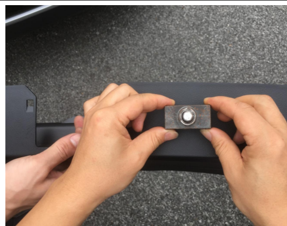
29. Use the hole opener to open the hole.
