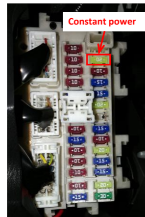
24. Location of the constant power fuse (first in the second column).
