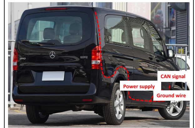
21. Route the power harness as indicated (if you need to install the added front switch, route the switch wiring harness in the same way).
