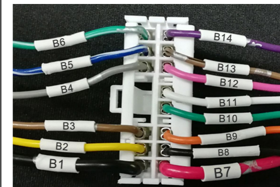
15. Insert the lock signal harness terminals into the wiring harness connector according to the diagram. Note: For models with fewer than 14 wires, just insert them according to the corresponding label or color.
