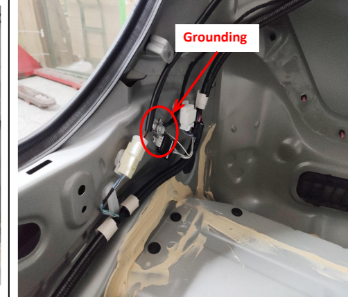
32. Ground at the indicated position on the left side of the trunk.
