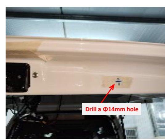
29. Drill a hole at the indicated location with a Φ14mm drill bit.
