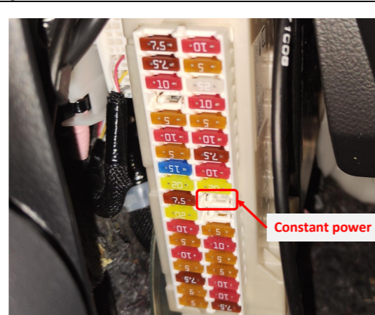
24. The fuse box is located at the driver's position and the fuse slot for power supply is indicated above.
