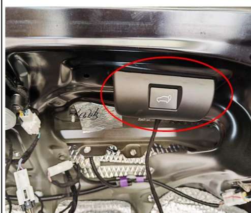
23. Install the added tailgate switch with the original screws.
