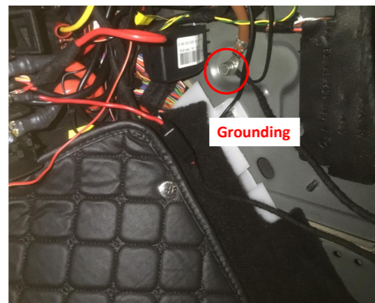
23. Ground at the lower right side of front passenger seat.
