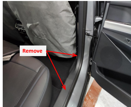
2. Remove the rear right side door sill panels and B-pillar trim panel.
