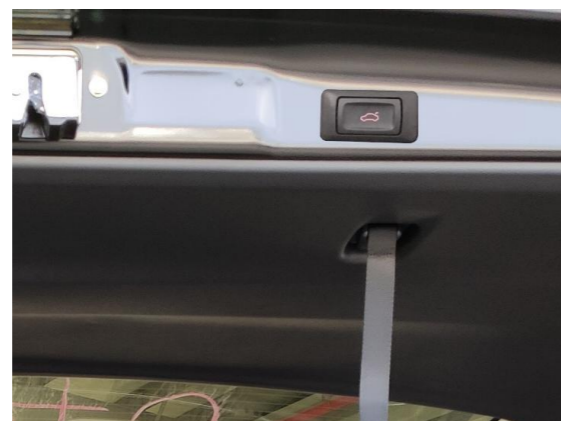
33. Reinstall all the trim panels and fit the added tailgate switch in.
