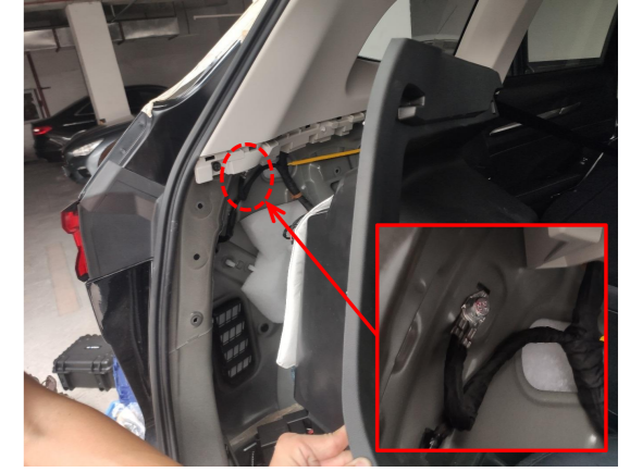
21. Ground at the left side of the trunk.
