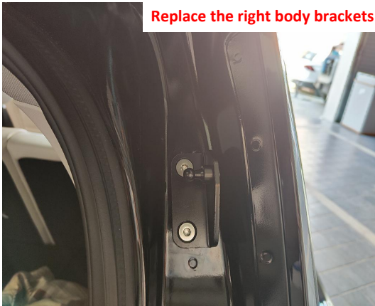
7. Replace the right body brackets
