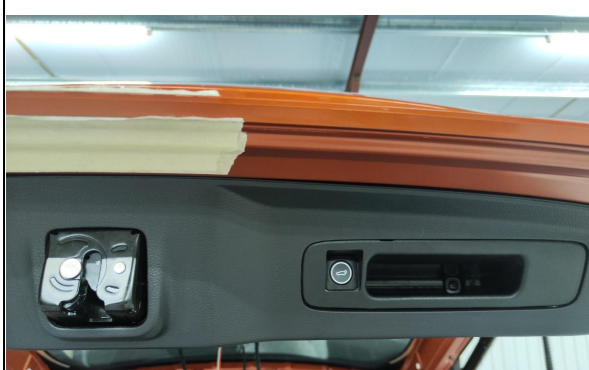
27. Install the added tailgate switch (remove the original handle) and Reinstall all the trim panels.
