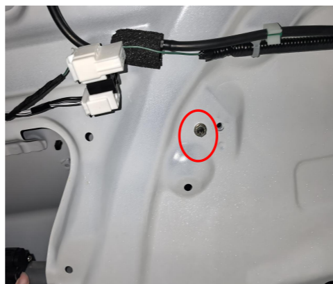
35. Fit the ECU into its bracket and tie the wiring harnesses to the original wiring harnesses.
