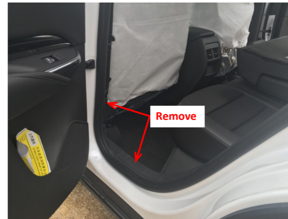
4. Remove the rear left side door sill panel and B-pillar trim panel.
