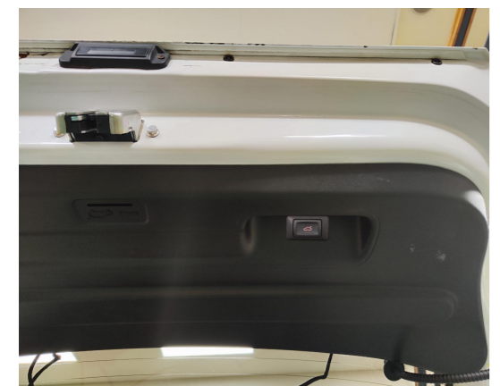
27. Install the added tailgate switch and reinstall all the trim panels.
