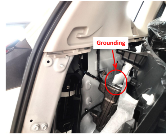
20. Ground at the left side of the trunk.
