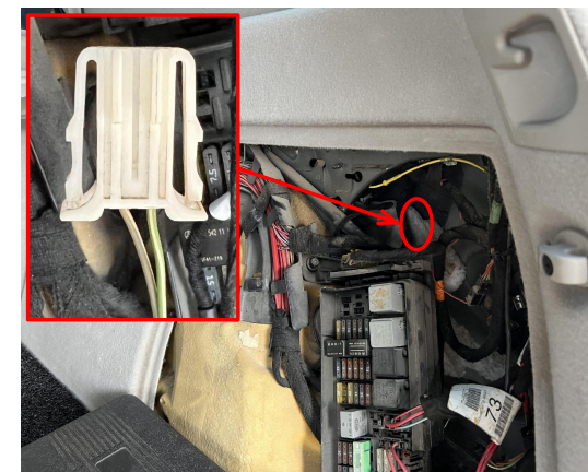
13. Connect the plugs of power harness to the plugs of unlock signal behind the fuse box.
