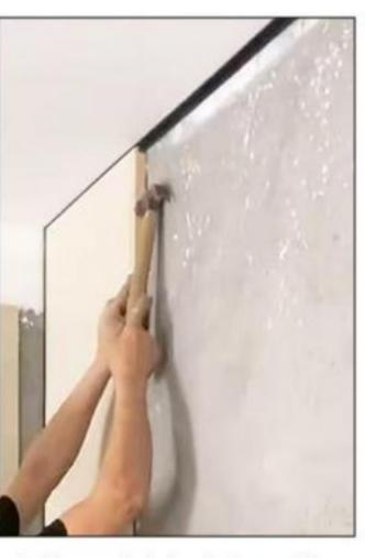
4. Close joint strike with a hammer to make the wall panels fit tightly.
