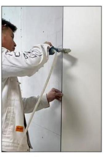
5. Fixed with brads install metal clips on the idle side and fix them with a brad.
