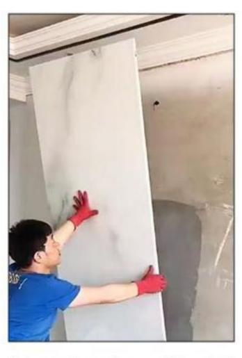
3.Install on the wall install the wall panels in sequence, align the male and female clips, and connect them to the wall.
