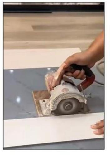
1.Wall panel cutting measure the size as needed cut with a handsaw.
