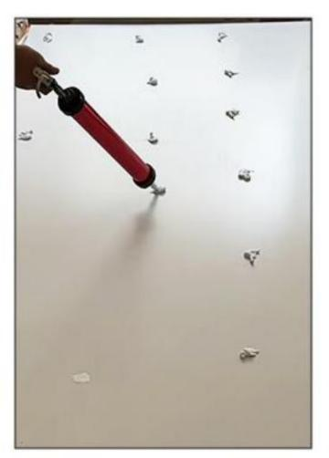
2. Apply adhesive on the back apply structural adhesive evenly on the back of the wall panel.
