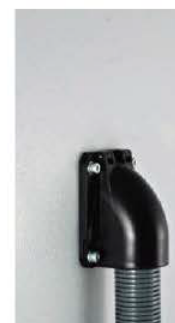
3. Lock FWS with screws
