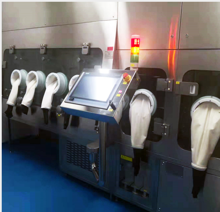
Class A Biological Safety Cabinet GMP construction environment: Class A biosafety cabinet in Class C clean area
