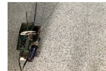
开槽焊接 Slot welding
