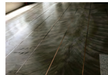
铺设铜箔 Laying copper foil
