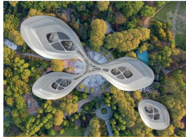
PV System Project Hainan, China | Year: 2019
