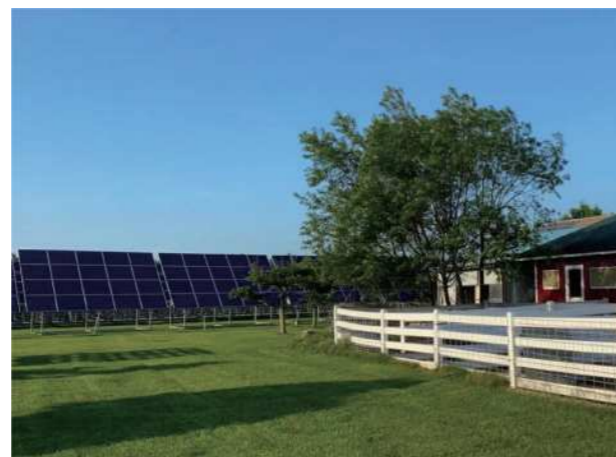
PV System Project Hokkaido, Japan | Year: 2022
